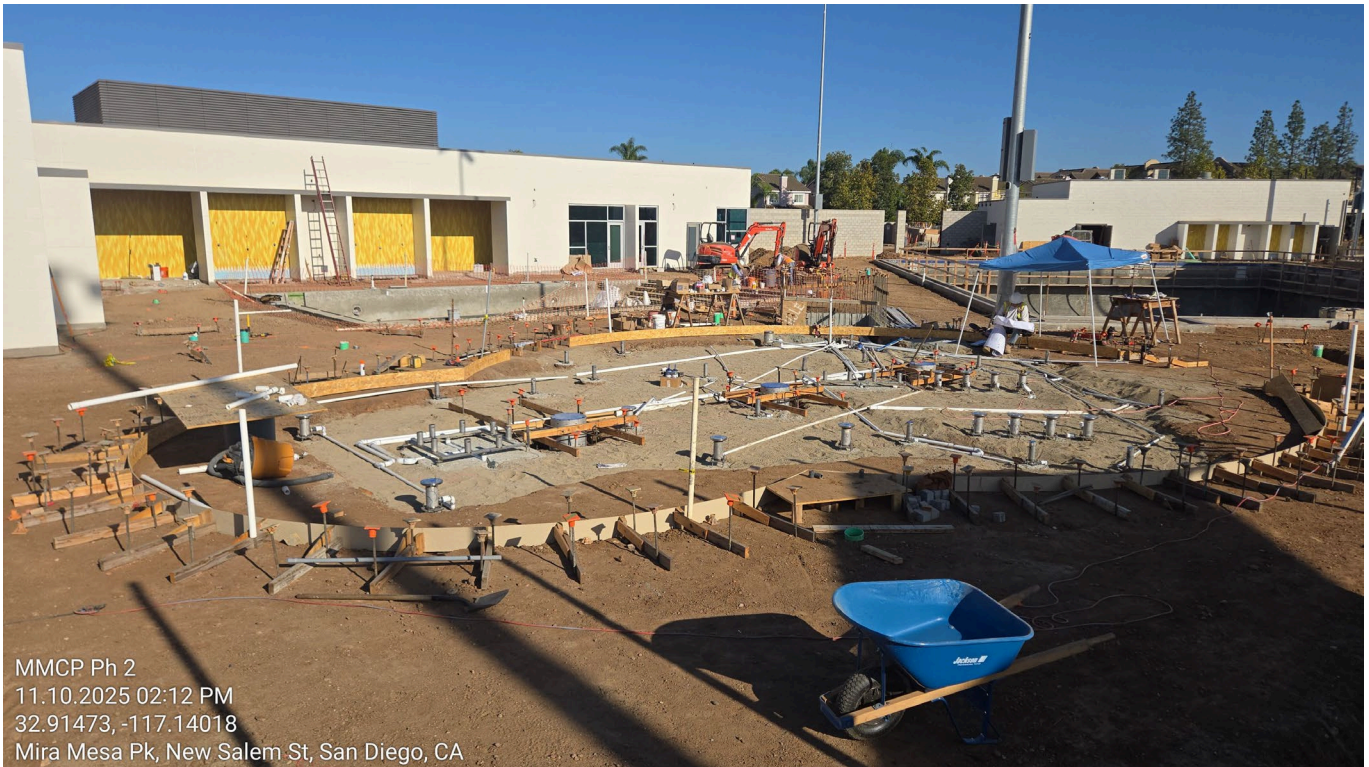
Installation of foundations and subgrade for wetplay toys
