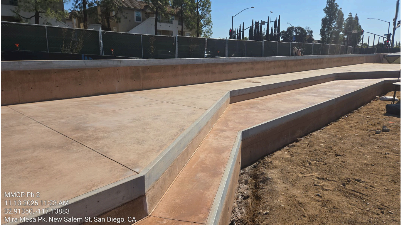
Installation of foundations and subgrade for wetplay toys
